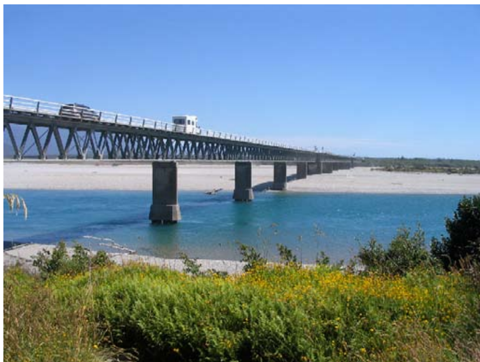
Haast road bridge, with two passing bays.
