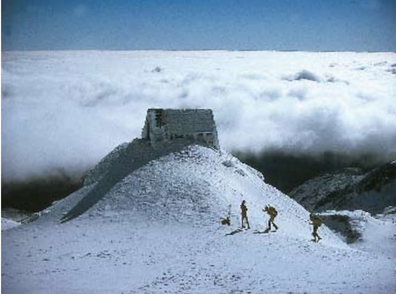
Winter photo of Dome Shelter, Mt Ruapehu (about 1981).
